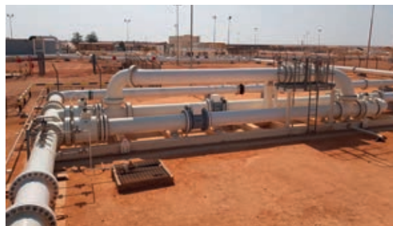
Custody transfer metering systems for produced water
