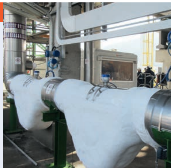
Custody transfer flow measurement for a bidirectional natural gas border metering station
