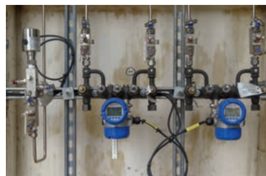
Pressure transmitter at a biomass plant
