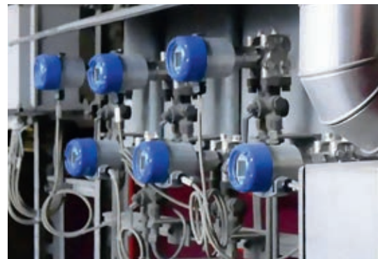
OPTIBAR DP 7060 differential pressure transmitters at a power plant
