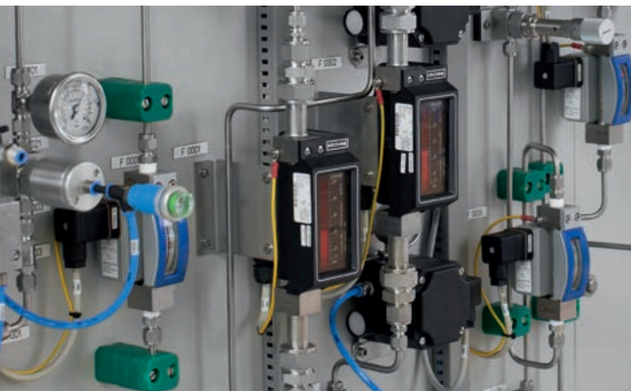
Measurement of sample flows in an analyser system
