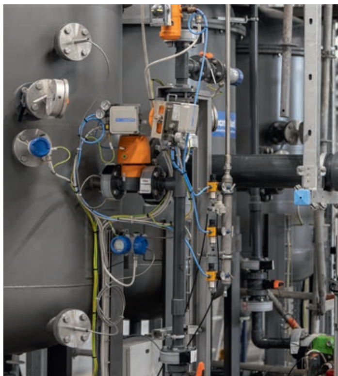
Level measurement in pressurised vessel
