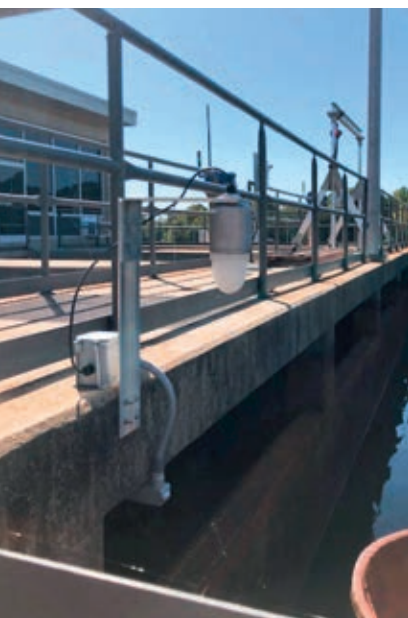
Radar level measurement of water basin
