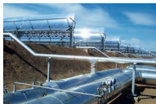
Flow measurement of thermal oil in a concentrated solar power plant
